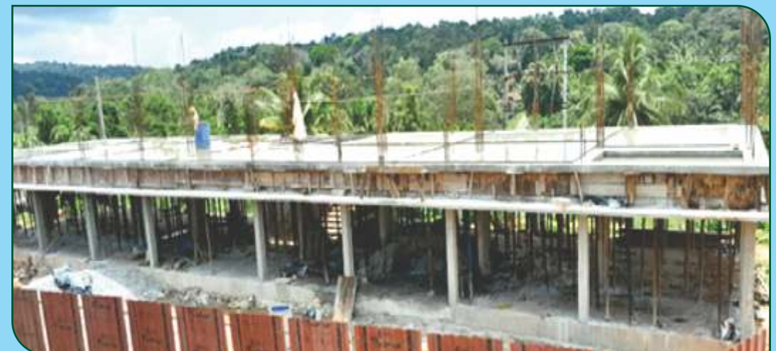
New building being constructed thanks to our 3 donors
